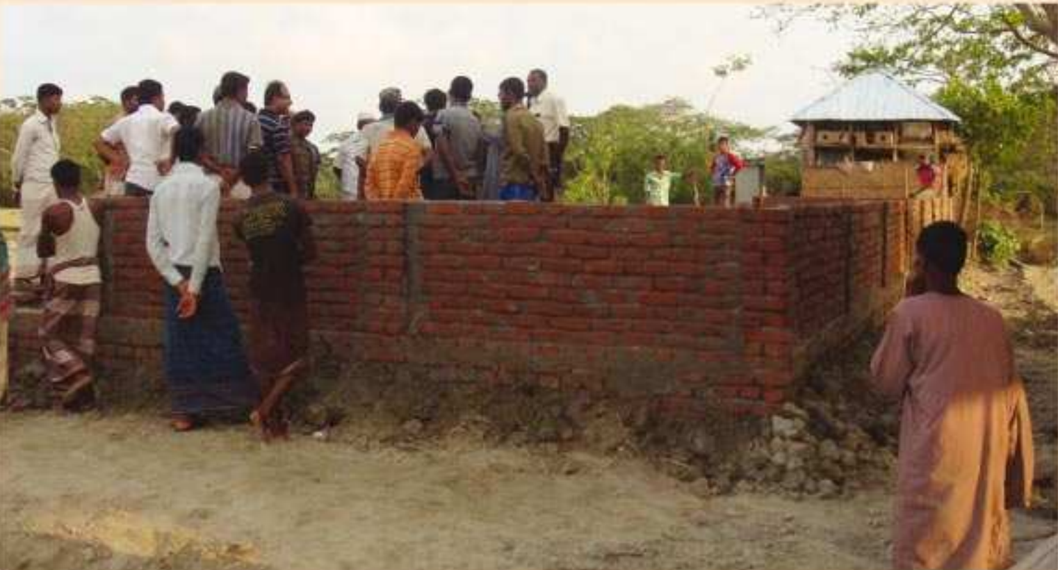
Construction of Sharifpara school building
