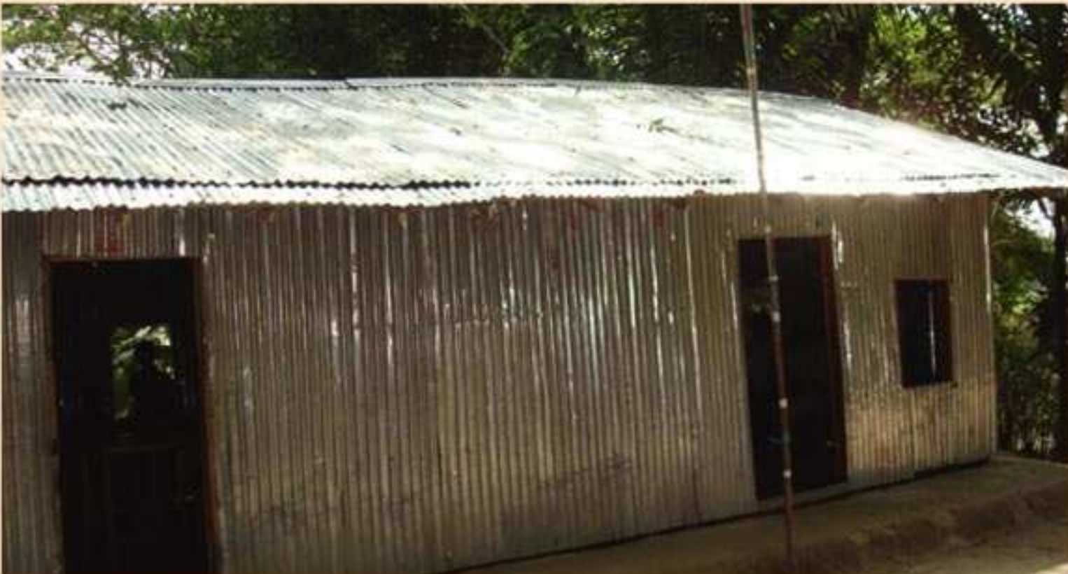
Renovation of Moddho Char Monohor school house
