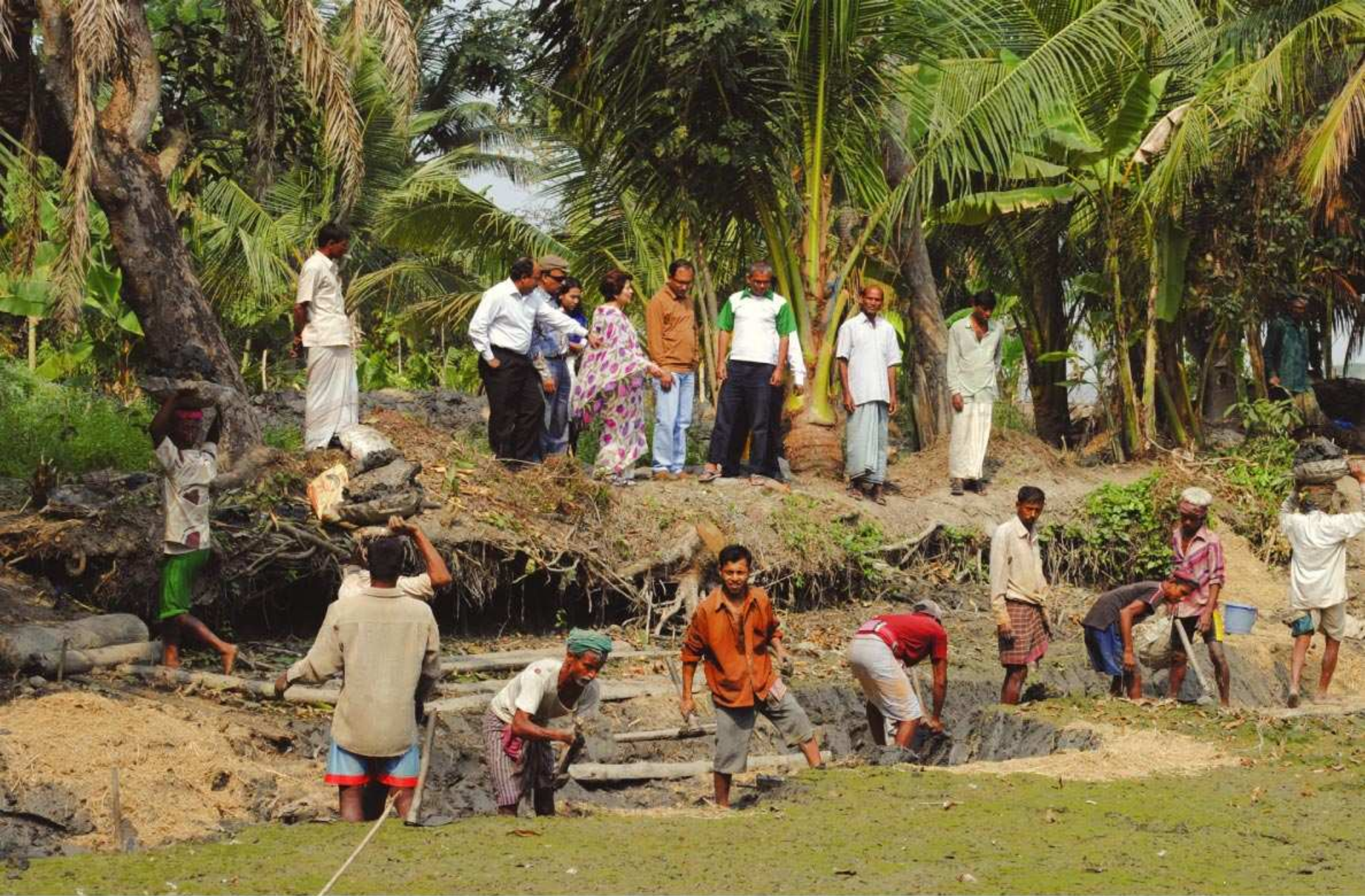
Pond re-exavation at Bon Laudob
